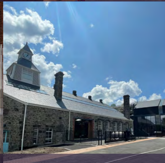
Wales Hafod Morfa Copperworks Redevelopment
