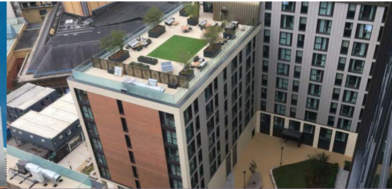
New York Square, SOYO, Leeds Y&H Caddick Construction, Moda Living, Burohappold Engineering, Richard Boothroyd & Associates Limited, DLG Architects, Tate Consulting
