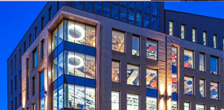
One Strawberry Lane North East Ask Real Estate Ltd, BAM Construction North East, Home Group, Ryder Architecture, AtkinsRealis, BGP Consulting Engineers, Shaw Construction Management, SES Engineering Services
