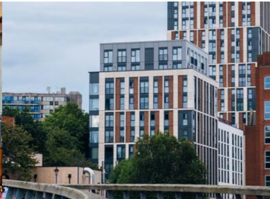
Castle Park View South West Bouygues UK, Linkcity with M&G Estates, Abri Homes, Homes England and Bristol City Council, Chapman Taylor Associates, Arup
