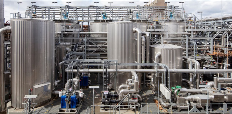
The Lostock Sustainable Energy Plant Enabling Works
