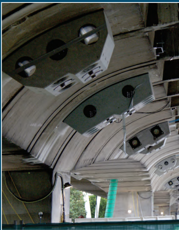
The blisters insitu prior to cable installation
