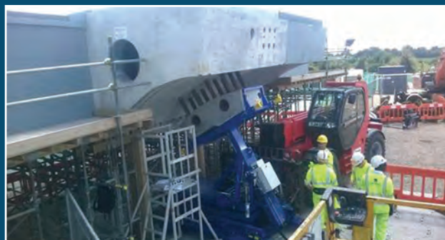
Blister installation at the mock up site
