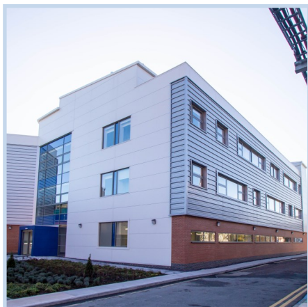
Catalyst Research Laboratory and Office Facility, Billingham, Tees Valley – National Winner of the Integration & Collaborative Working Award 2014
