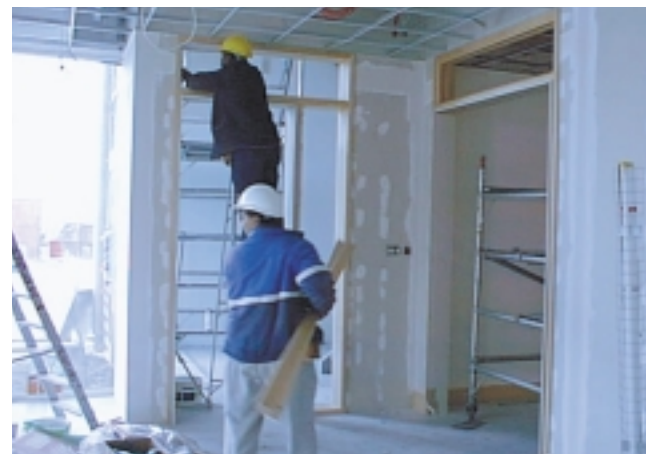
Fit-out at Meggitt Mobrey, Slough
