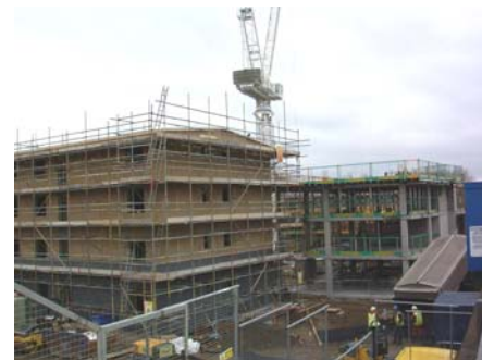
Access to main site storage area blocked during site operations
