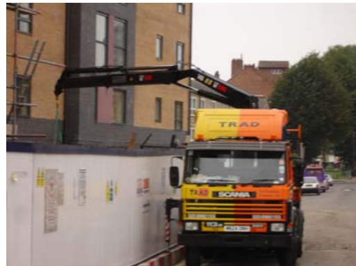
HIAB being used to collect scaffolding from behind the site hoarding
