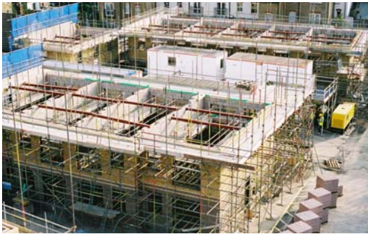
Blocks off-loaded into temporary holding areas
