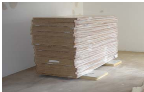
Doors placed in a central storage area on the appropriate floor
