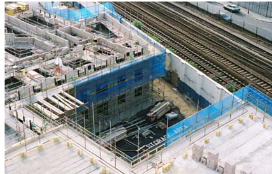
Blocks loaded out ready for laying
