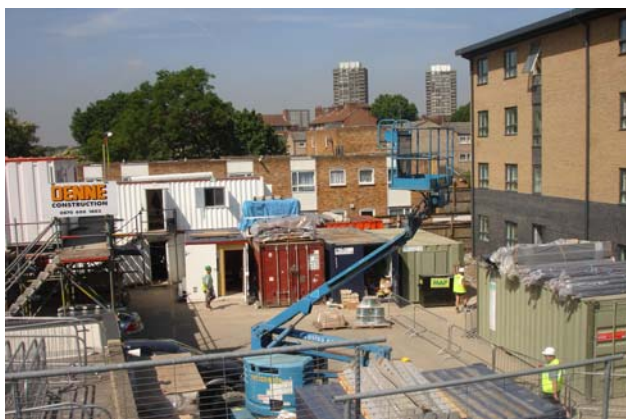
Central storage area on Talwin Street accessible by forklift.
