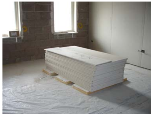
Plasterboard stacked ready for fixing
