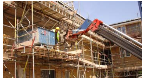
Forklift removing a rollover-tipping bin from 3rd storey loading bay
