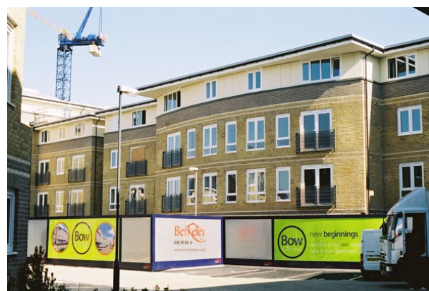
Block B nearing completion
