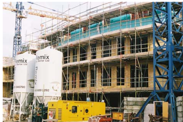
Block B of the Ordell Road scheme under construction
