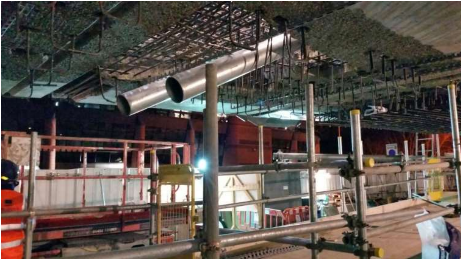
Long tendon anchorage works
