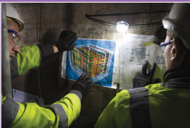
Figure 9: 3D modelling assisting with reinforcement fixing
