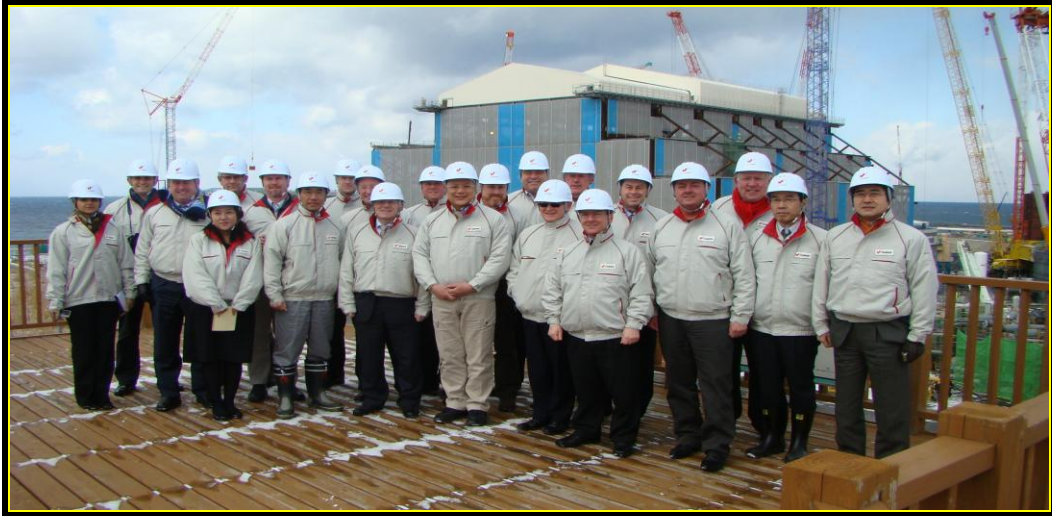
The tour party with our hosts at the Ohma nuclear power station under construction
