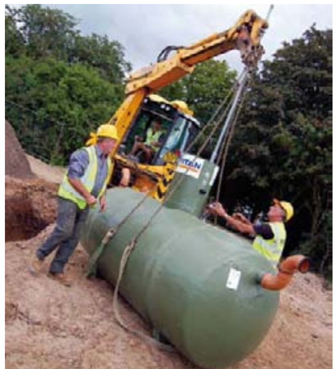
Installation of the rainwater harvesting tank
