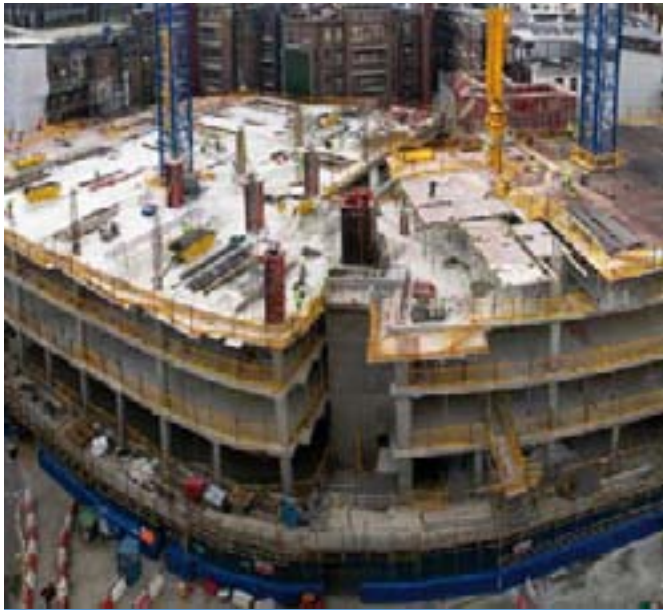
Barts site March 2008
