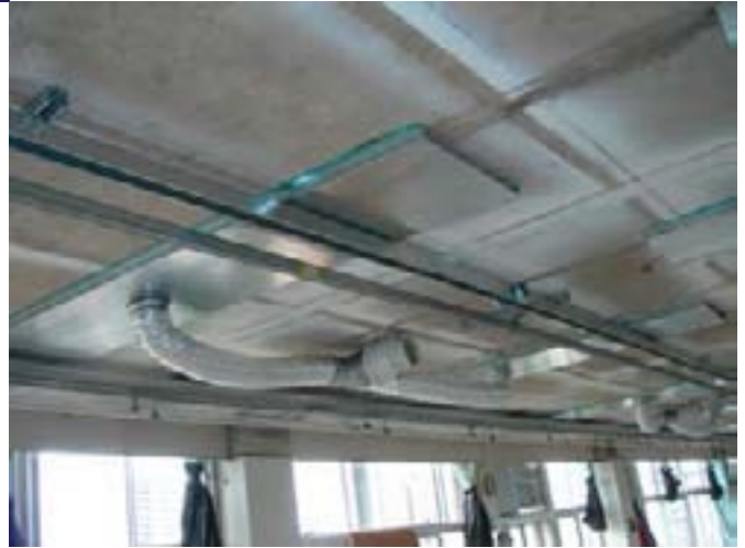
CoolDeck being installed
