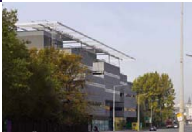
The roof rack design of the PV array provides solar shading for the glass atrium, reducing the need for mechanical cooling
