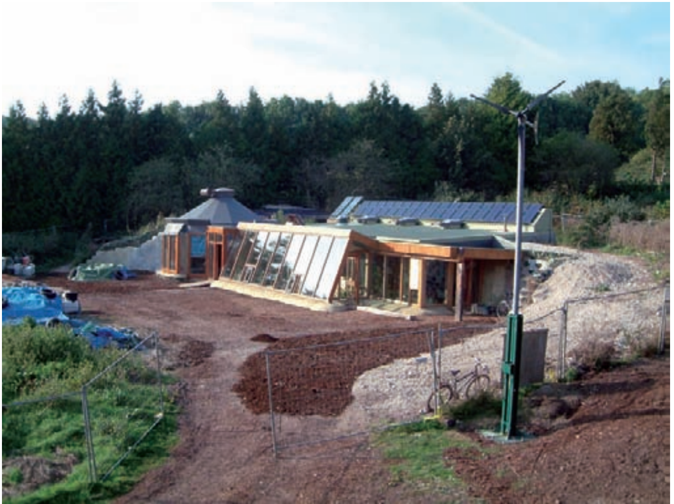
Earthship Brighton during construction
