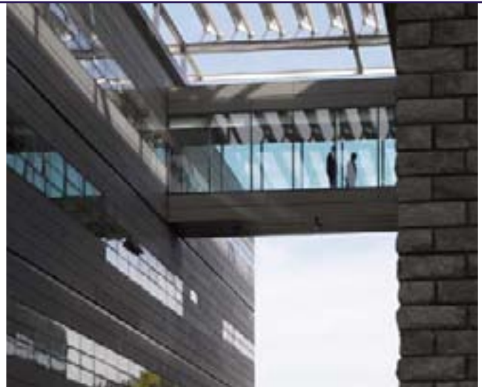
The enclosed bridge over the newly created pedestrian walkway
