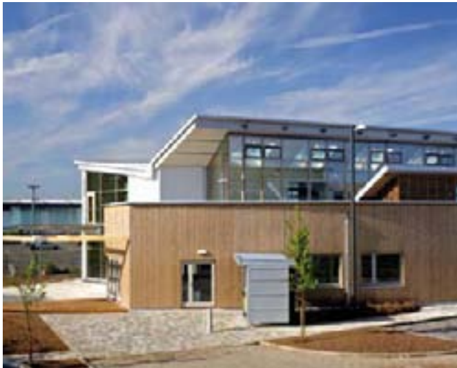
SBC completed in April 2008
