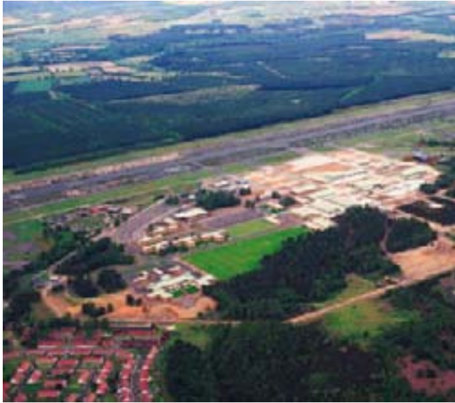
Aerial view of Woodbridge Airfield
