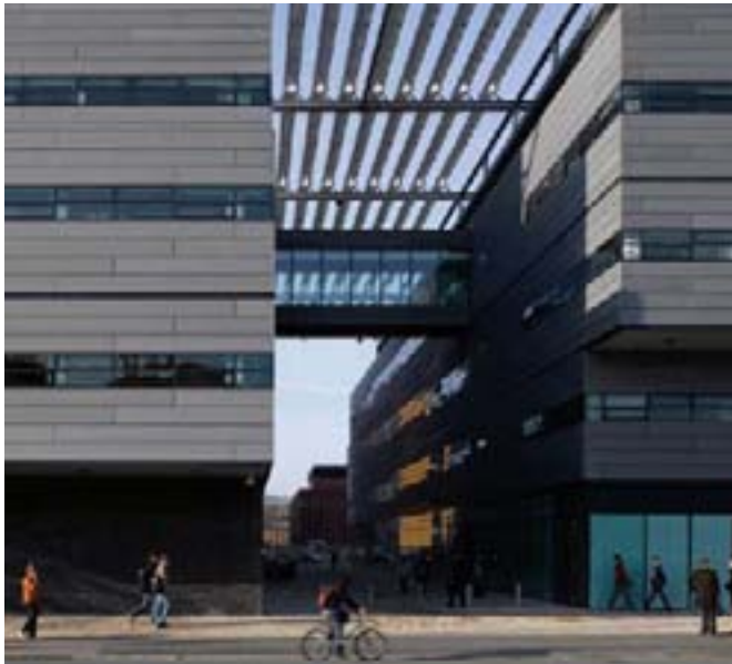
The PV array is mounted on 100 steel frames which sit across the top of the building (as seen here)
